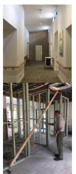
Despite the cold and sometimes very wet days, we have been busy getting ready to renovate the end of our Yellow Wing. The end of the corridor to the wing has been sealed off (sec Pictures left) and we are at framing stage to add 3 more rooms under the roofline.
